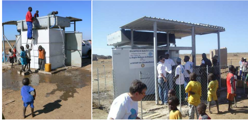
FIGURE 4. INSTALLATION DE LA STATION HYDROPUR EN 2009
